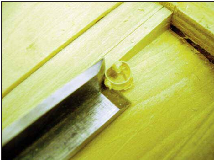
Figure 92. Corner chisel in use.
