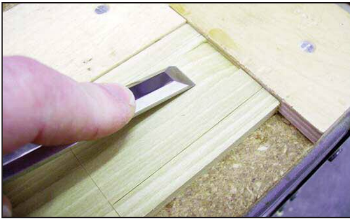
Figure 90 (above). Waste material of chamfer is removed with a chisel.
